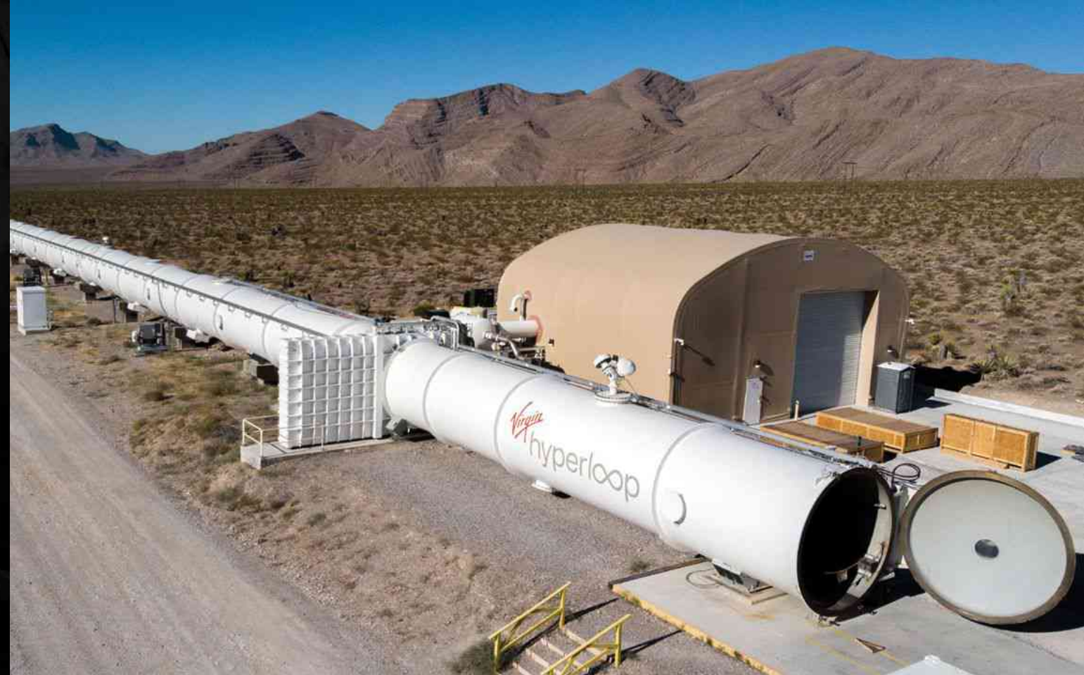
▲ Nevada, USA Hyperloop One's 500-meter Development Loop (DevLoop). Photo: Virgin Hyperloop One.
