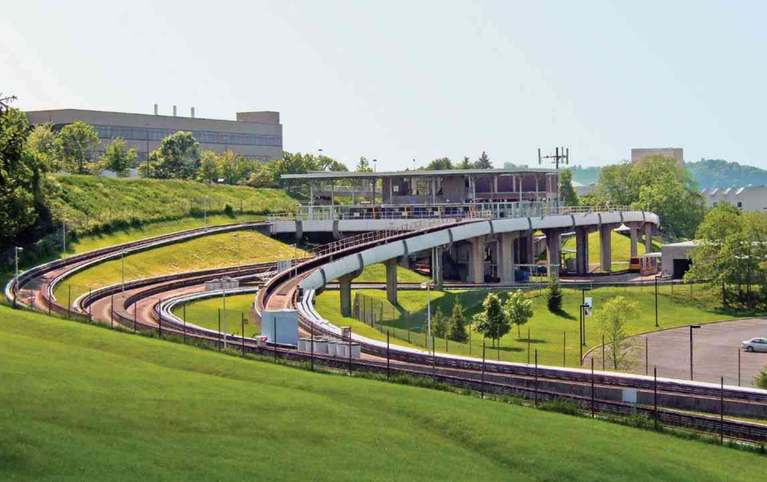
▼ Morgantown, USA America's one and only personal rapid transit (PRT) system connects the three Morgantown campuses of West Virginia University and the city's downtown area. The driverless system was a government-funded experiment which opened in 1975. Like all PRT systems, stations are built on sidings, which allows vehicles to bypass stations and enables express trips between any two station pairs. Photo: Jae69376 (above), Antony-22 (below)
