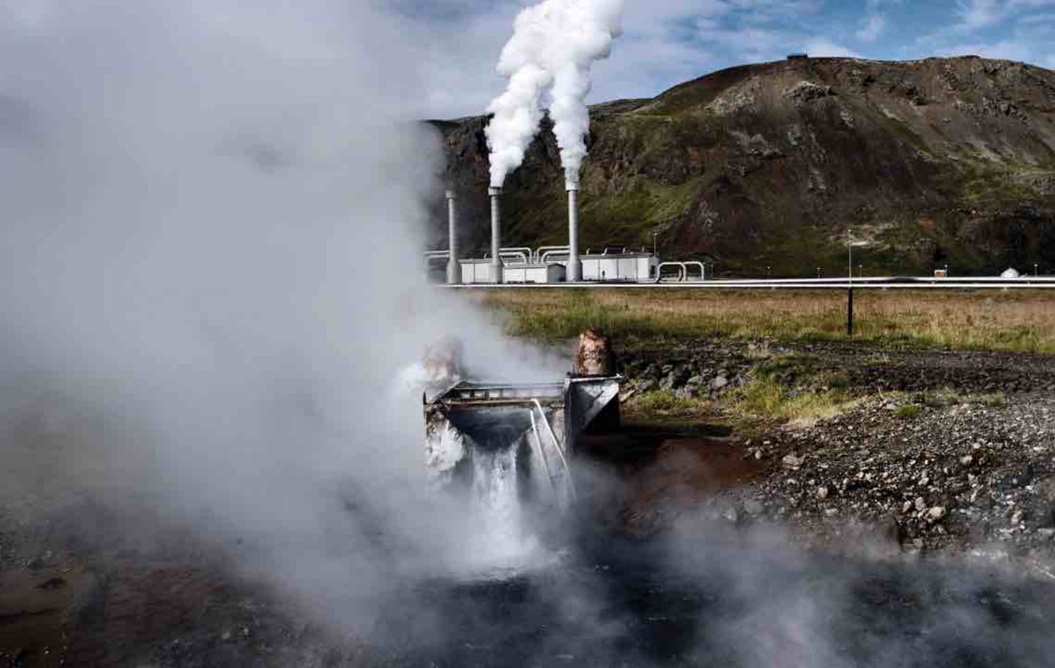
▲ Hengill Nesjavellir geothermal plant generates electricity and hot water by utilizing geothermal water and steam.
