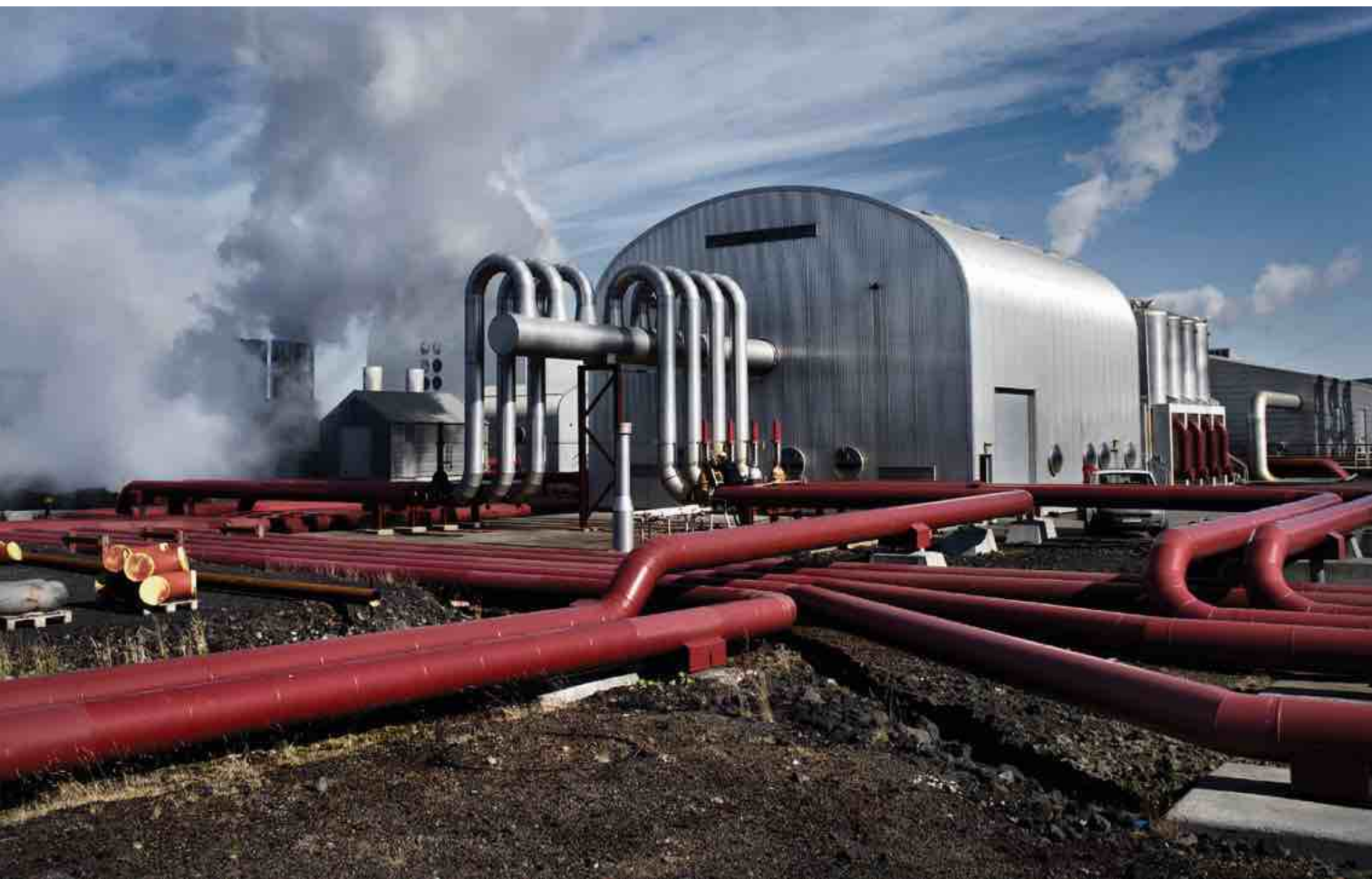
▲ Hengill Nesjavellir geothermal plant generates electricity and hot water by utilizing geothermal water and steam.
