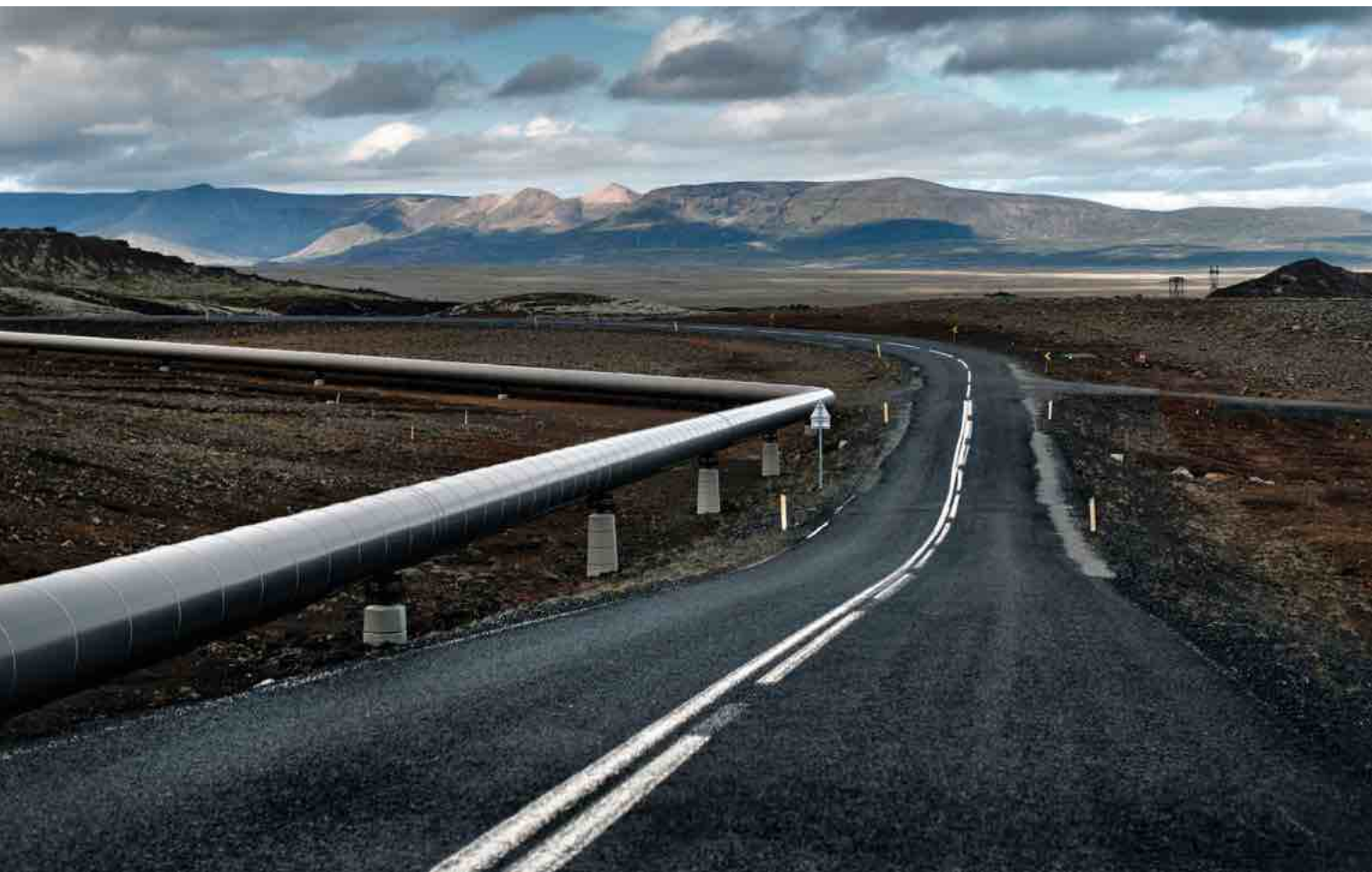
▼ Hengill On the road from Hellisheidi Power plant to Reykjavik, city pipes carry hot water to be used for heating.
