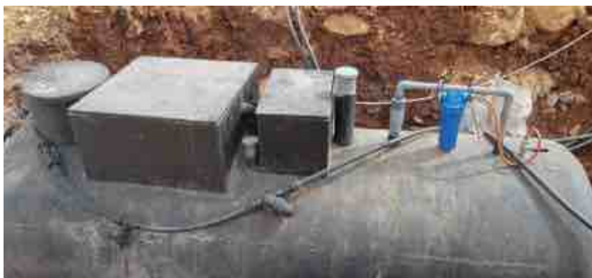
1. & 2. The CubeX could be installed in the vicinity of a dwelling and could treat all bio-wastes and recover cooking gas, irrigation water and compost.
