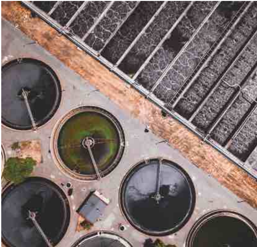
7. Water filtration ponds. Photo: Ivan Bandura
