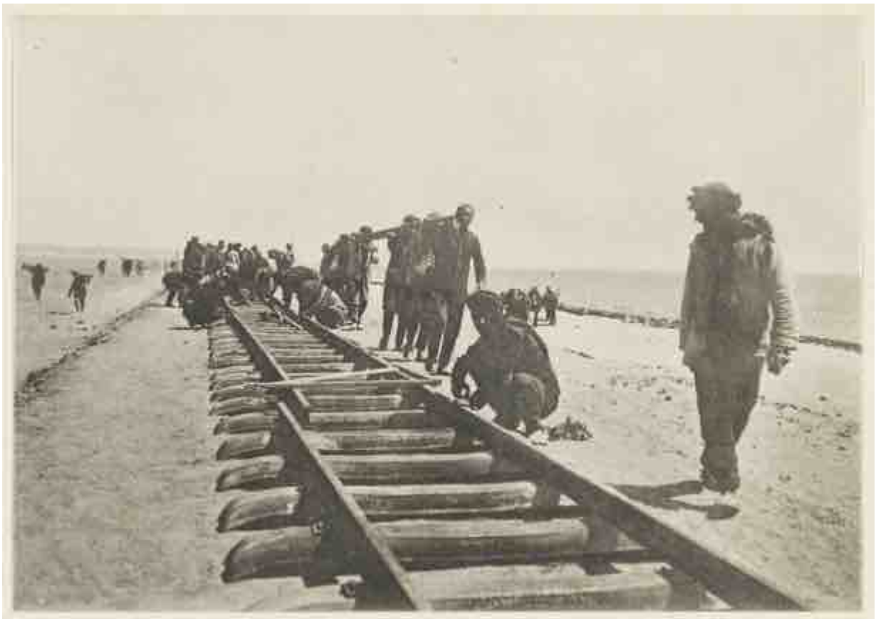
▲ PUTTING THE RAILS FOR THE CONSTRUCTION OF THE HICAZBAHN AT TEBUK, 1906. SOURCE: BERNHARD MORITZ
