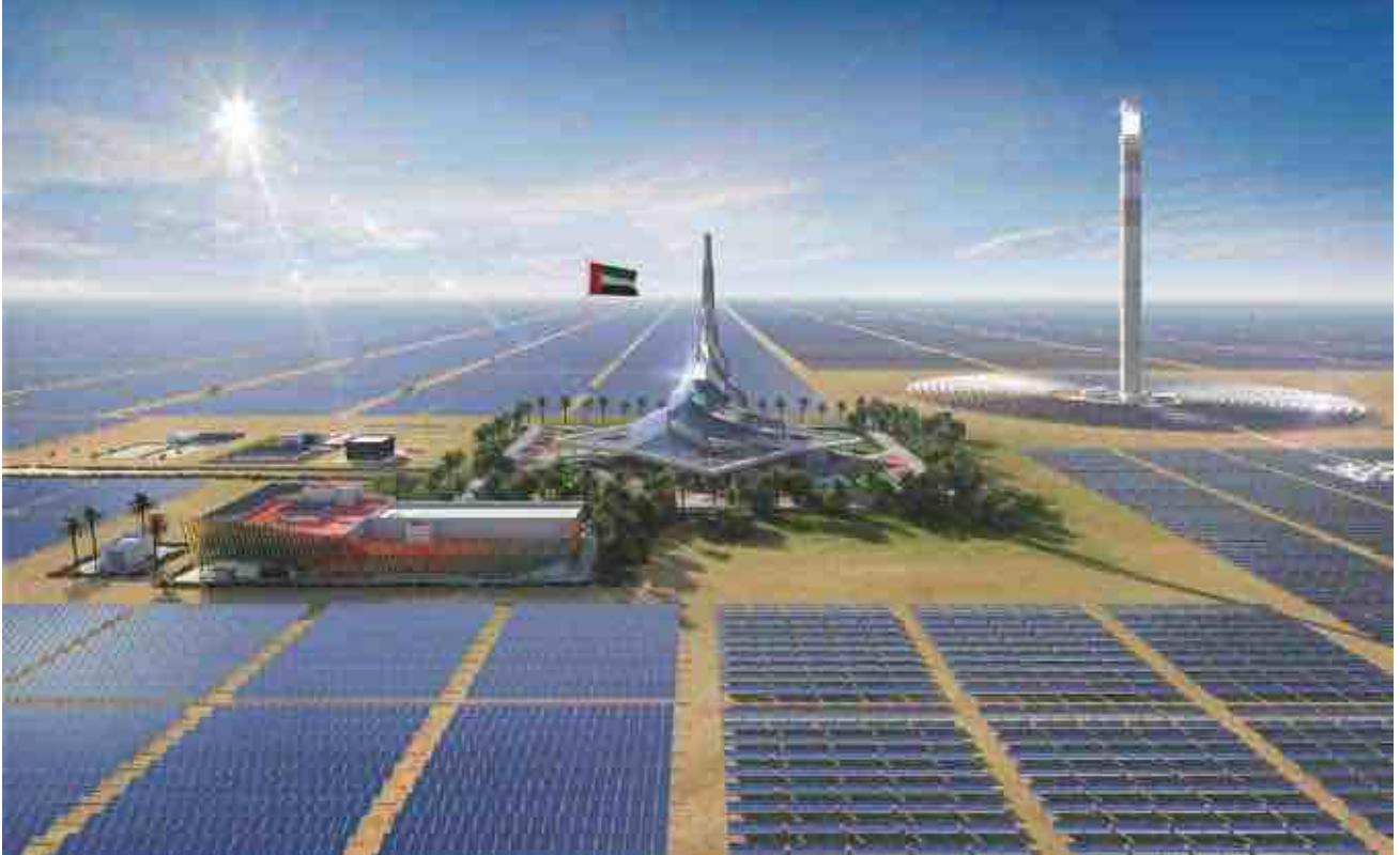
▲ THE 5GW MOHAMMED BIN RASHID AL MAKTOUM SOLAR PARK, CONTAINING THE BIGGEST CONCENTRATED SOLAR POWER (CSP) PROJECT IN THE WORLD (700 MW).
