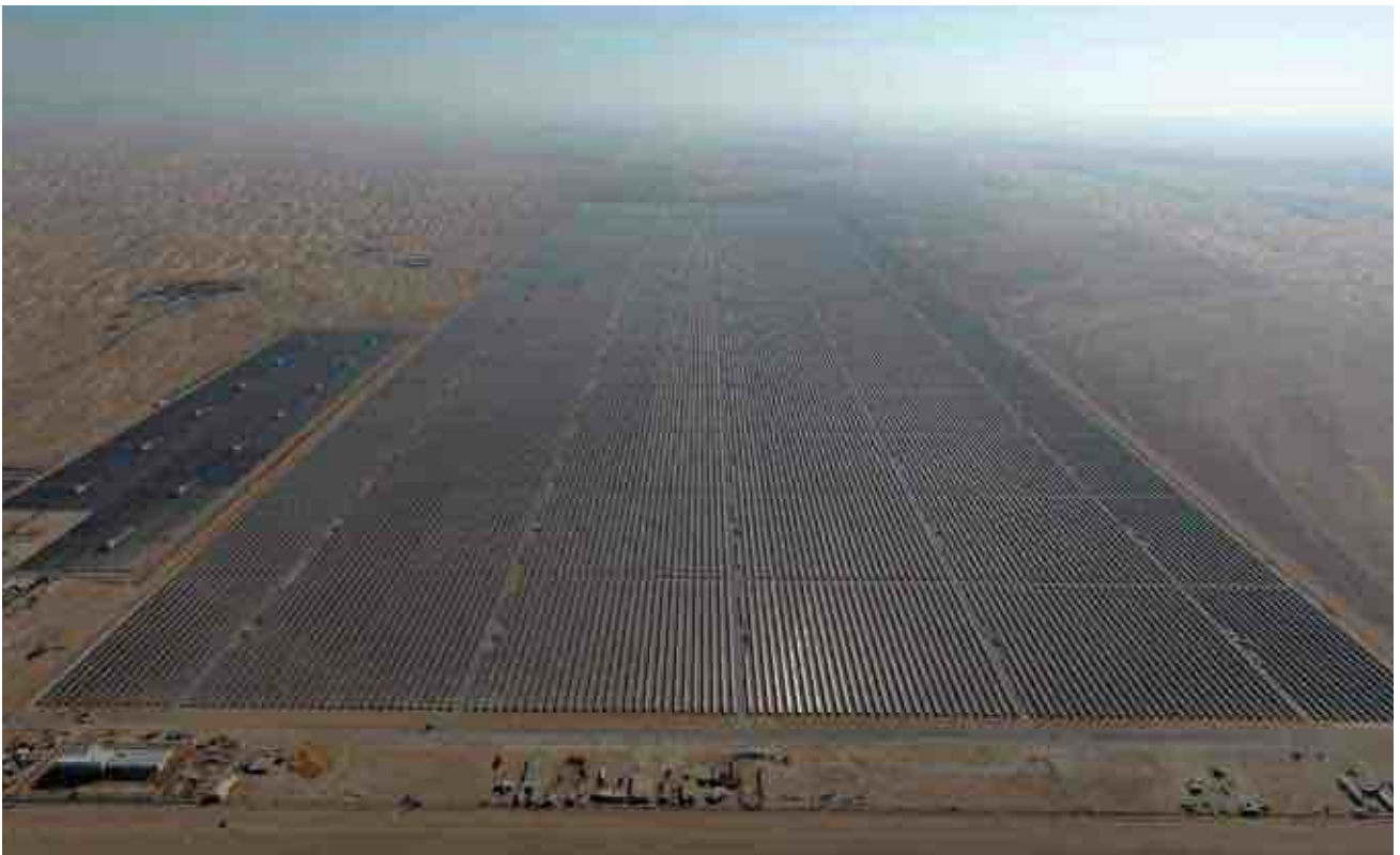
▲ THE CONSTRUCTION OF PHASE II OF THE 5GW MOHAMMED BIN RASHID AL MAKTOUM SOLAR PARK AS COMPLETED IN 2017.
