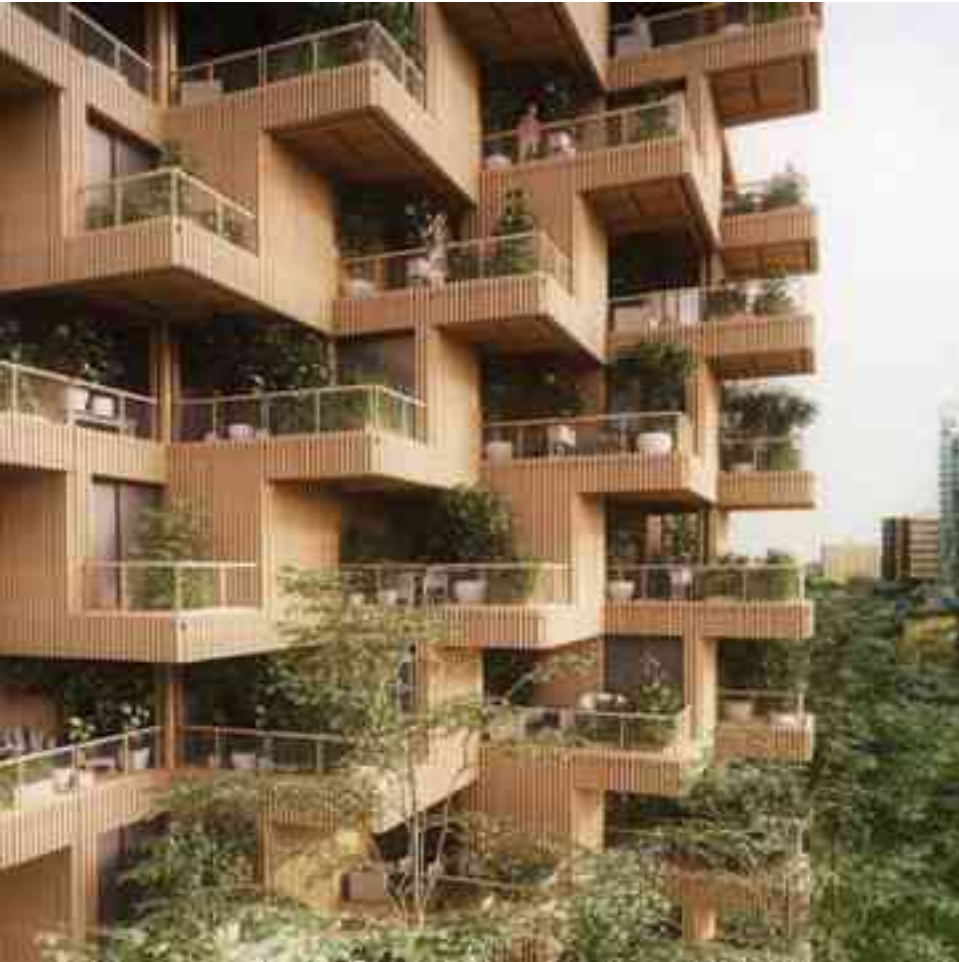
PLANTS AND TREES SPROUT FROM THE MODULAR UNITS THAT MAKE UP THIS TIMBER-FRAMED HIGH-RISE, PROPOSED BY ARCHITECTURE FIRM PENDA. THE TORONTO TREE TOWER IS BUILT FROM CROSSLAMINATED TIMBER MODULES.
