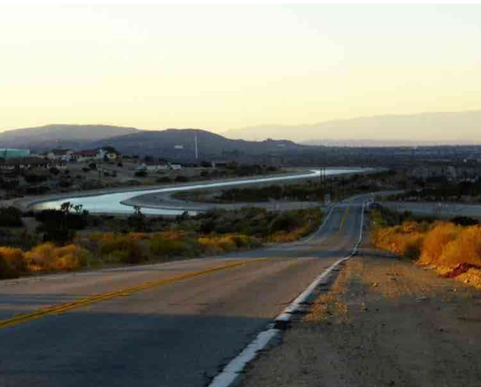
California Aqueduct Crossing the San Andreas Fault, USA Source: Michael R. Perry
