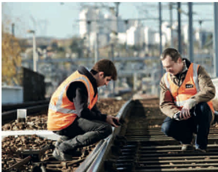
Checking the train network infrastructure. Source: Yann Audic / SNCF
