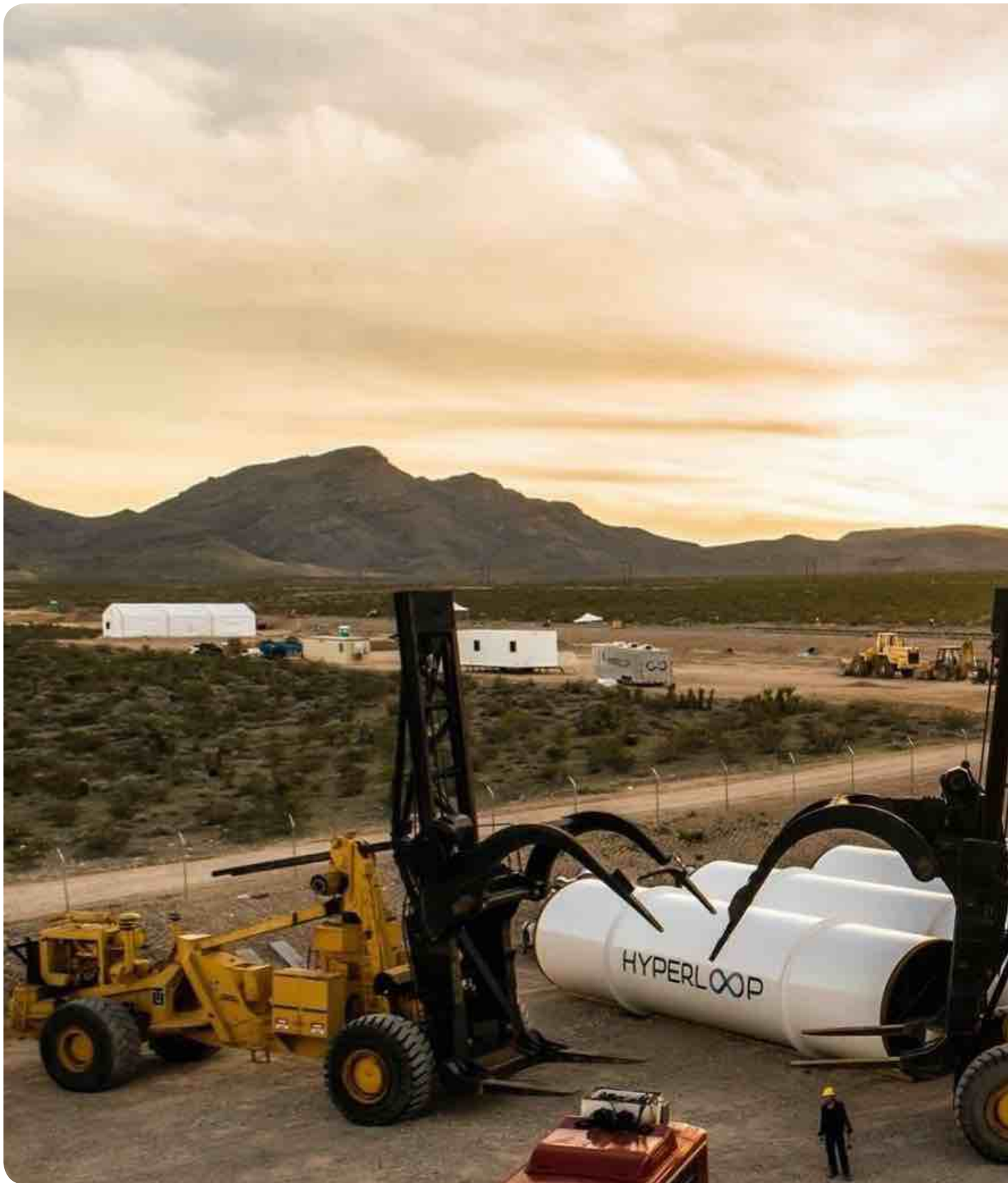
Construction site of a short 3 km test track in the Nevada desert to test lightweight prototype Hyperloop pods. Source: Neil Wood / Hyperloop One
