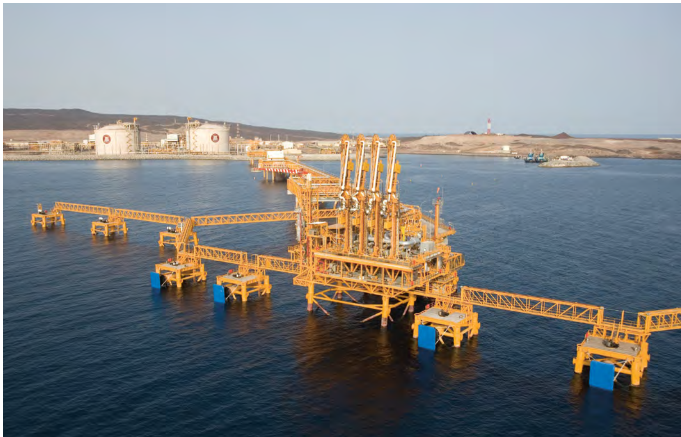
Jetty with loading arms of LNG factory, Balhaf, Yemen. Source: Thierry Gonzalez
