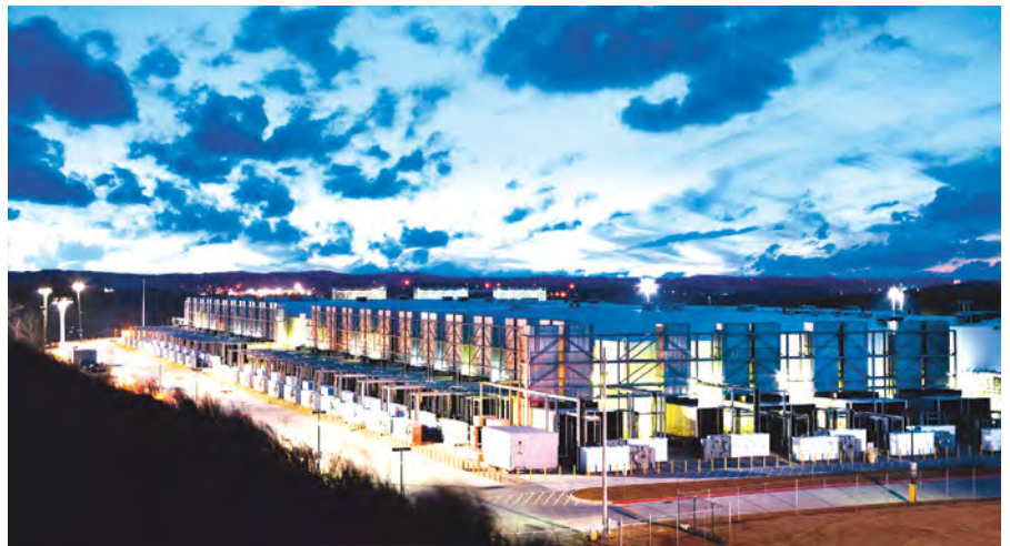
Google data center, Atlanta, Georgia. Source: Google.
