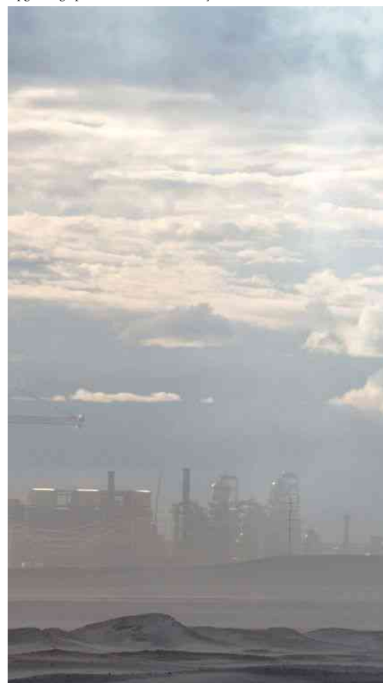
Upgrading operations, Fort McMurray
