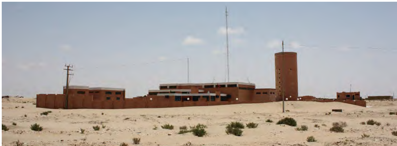
Desalination plant on the Saharan coastline, Tarfaya, 2010.
