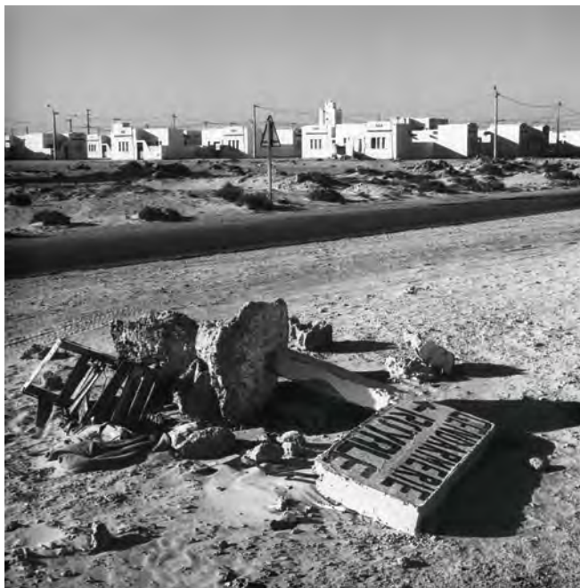
Deserted Moroccan development on the road between Layounne and Asmara.
