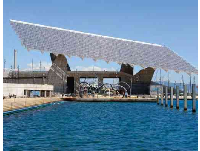
Solar photovoltaic plant provides energy to the city. Courtesy: Municipality of Barcelona.
