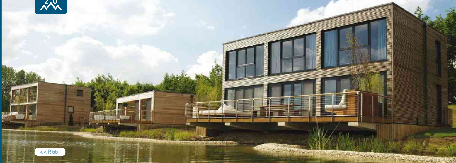
The Lakes Project (2007): 160 wooden family houses placed around six lakes in Cotswolds, Great Britain (160 km from London). Energy efficient villas are designed by architect Philippe Starck and Yoo Architects and built by Riko.
